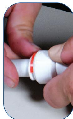
**NOTE: To identify hot and cold water circuits, red and blue collet clips can be fitted.**
