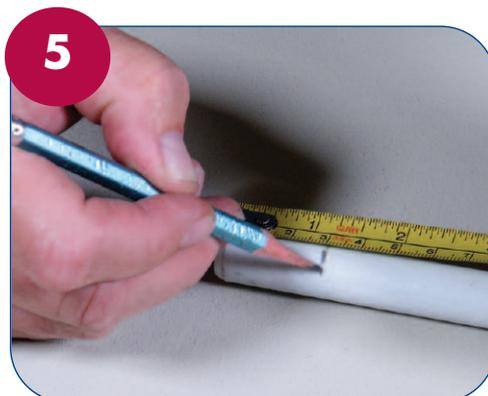
✓ Measure and mark the correct insertion depth on the pipe.
