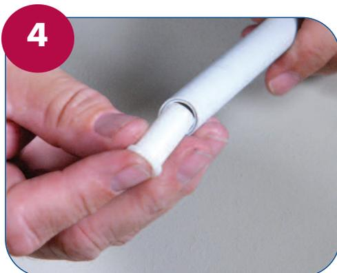
✓ Fit the correct insert into the pipe.
