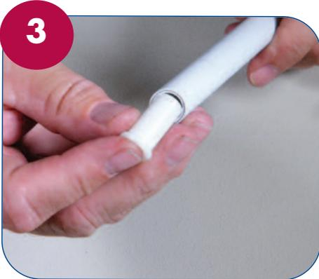
✓ Fit the insert into the pipe.
