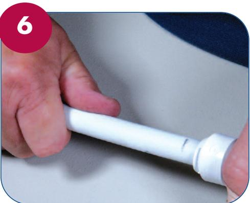
✓ Insert the pipe into the fitting, ensuring it passes through the O-Ring, until it reaches the stop point and correct insertion depth.
